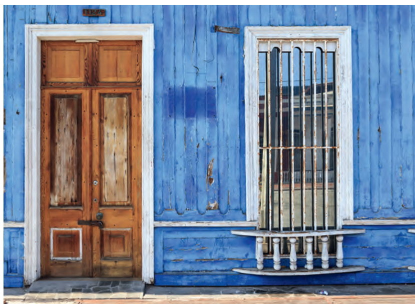
Fachada Casco Antiguo / Old Town Facade
